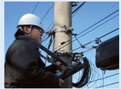
Splicing aerial drop cable
